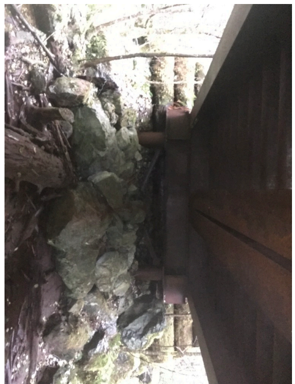
Left Bank Abutment when facing downstream
